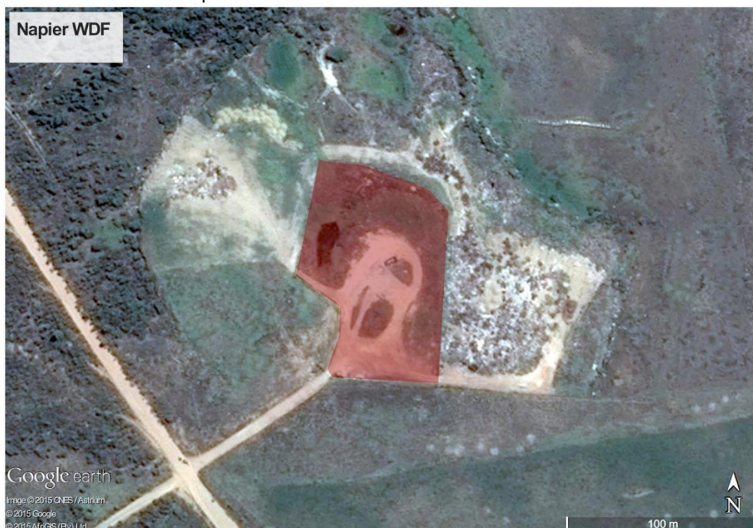
Figure 14 Napier Waste Drop-off Facility Site
