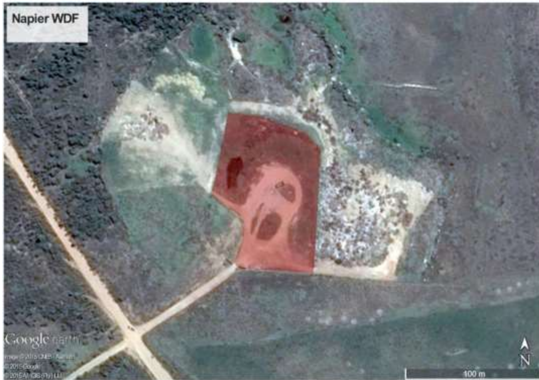
Figure 10. Napier Waste Drop-off Facility Site (Source: Google Earth)
