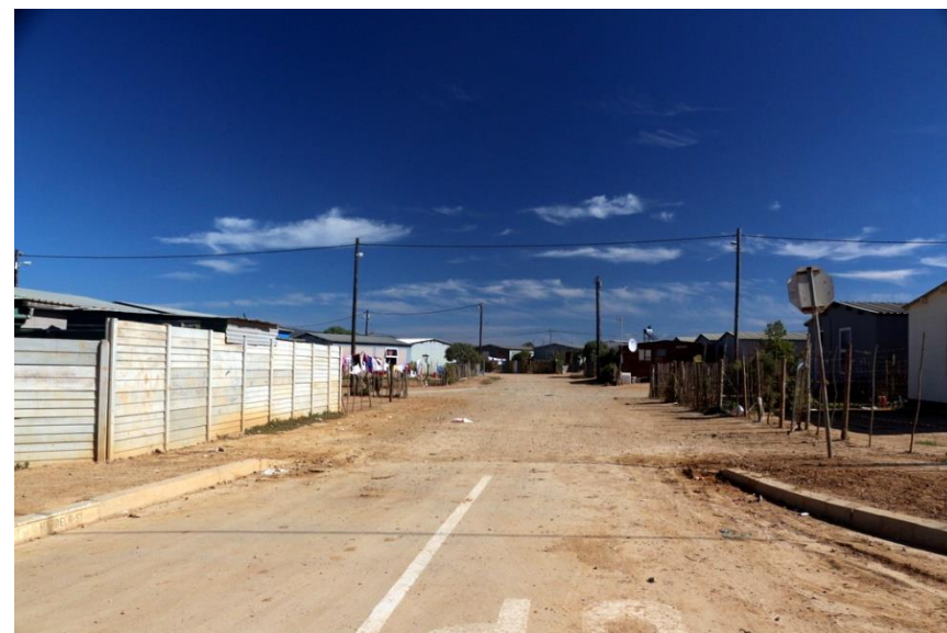
PHOTOGRAPH 6. SUBSIDISED HOUSING IN BREDASDORP
