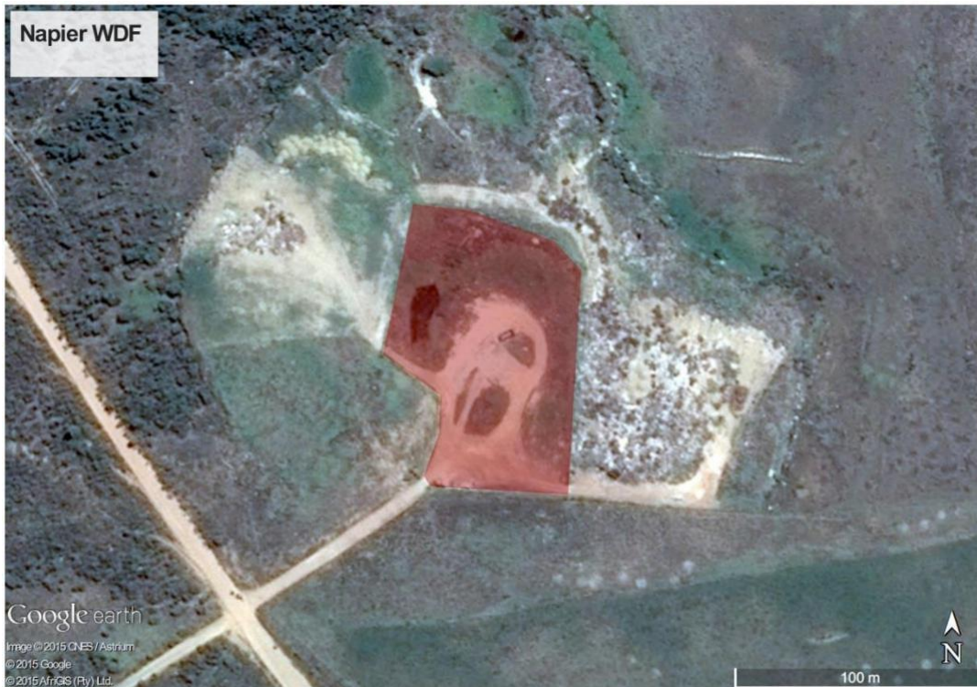
Figure 14 Napier Waste Drop-off Facility Site
